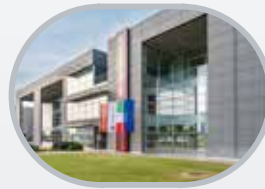
CAVRIAGO (RE) PRODUCTION AND NEW INNOVATION CENTER
